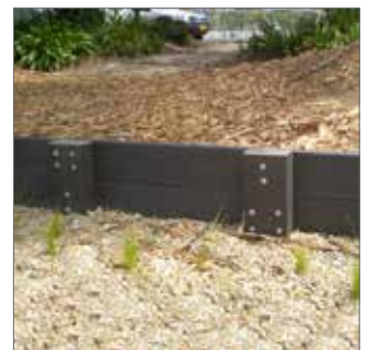
74752 Moodie Cat-Lyne Retaining Wall
