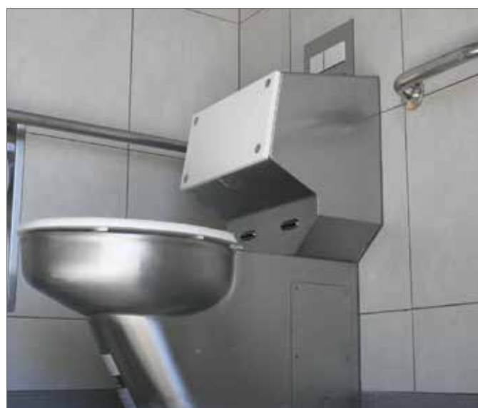
Toilet pan stainless steel. Note backrest and vents for air drying
