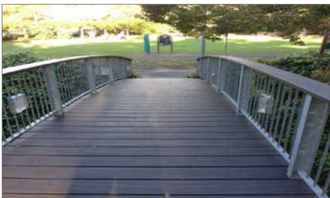
WILLOUGHBY COUNCIL - CHELSEA PETERSON 9777 7732 Muston Pk Bridge: Roocycle ET decking and Handrail
