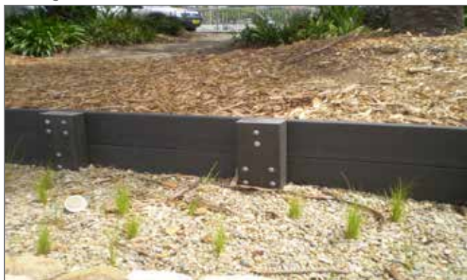
WOOLLAHRA COUNCIL - ROD WARD 9391 7060 "Catalina's" Car Park, Rose Bay: Roocycle ET Retaining Wall
