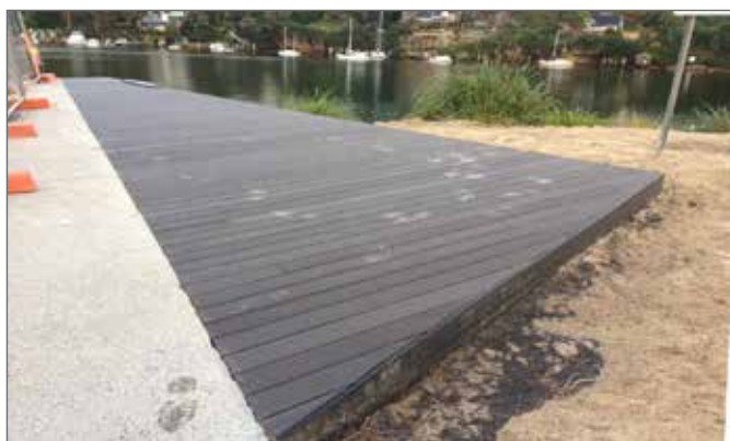
MOSMAN COUNCIL - JOHN GRADY 9978 4060 Ellery Pk, Spit Bridge: Roocycle ET substructure with Enviro Decking
