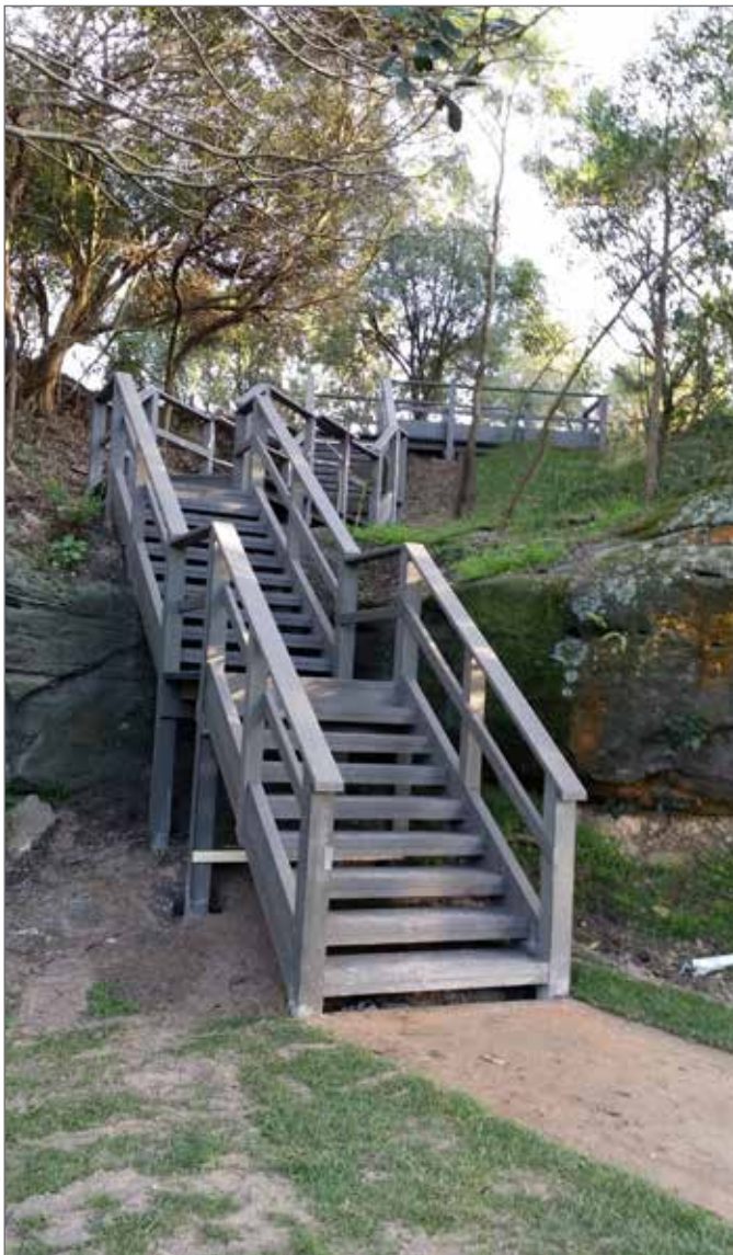
NORTH SYDNEY COUNCIL - DAVID BANBURY, 9936 8205 The Coal Loader Steps: Roocycle ET substructure, treads & handrails
