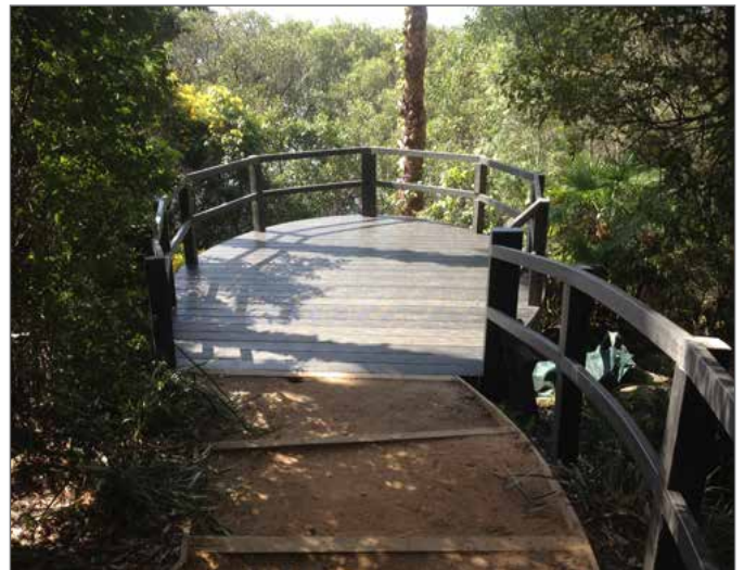
CANADA BAY COUNCIL - BEN RICHARDS, 9911 6335 Kokoda Track Viewing Platform: Roocycle ET substructure, decking & handrails
