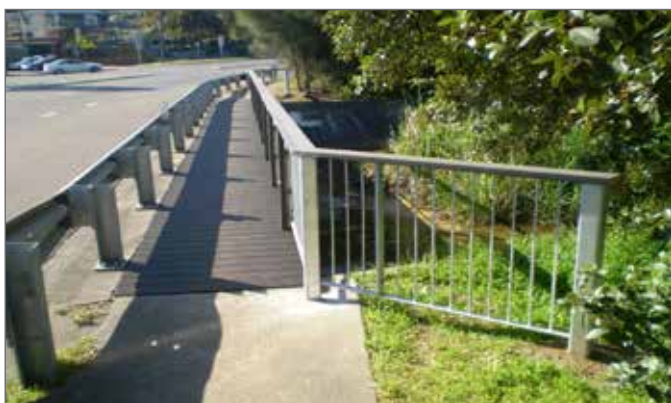
PITTWATER COUNCIL - GLYN AVEREY 0408 408 805 Avalon Pedestrian Bridge: Roocycle ET decking and handrail
